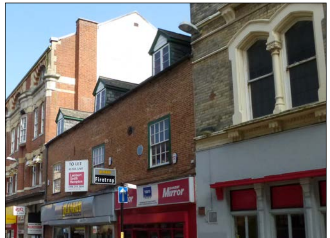
Good quality bricks laid in decorative patterns helps form a strong positive character for the area and contribute towards its local distinctiveness.
