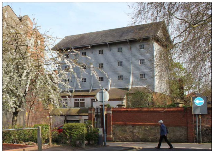
View of former timber-drying warehouse at rear of 66 Church Gate from Butt Close Lane.
