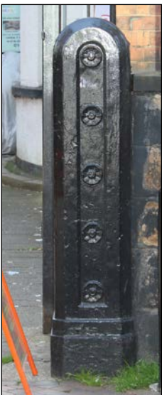
Cast Iron gate pier at 66 Church Gate.
