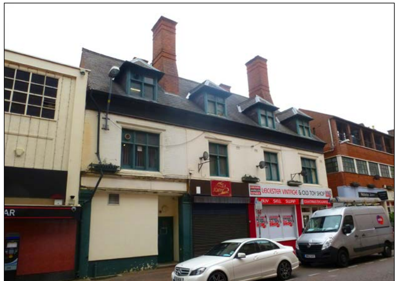
9-15 East Bond Street retains much original character including prominent chimney stacks and leaded glass – elements of the historic shopfronts survive beneath security features.
