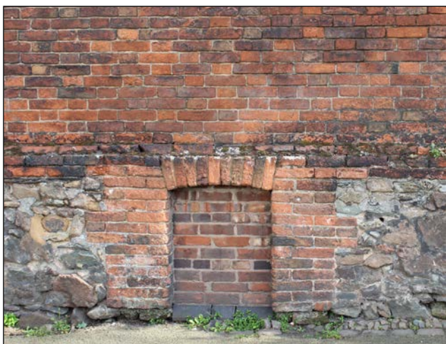
Brick and Stone detail: Butt Close Lane Wall
