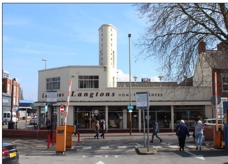
81 Church Gate is one of two former car garages in the area, the distinctive ‘fin’ forms an interesting corner feature
