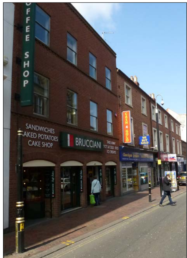
Upper floor adverts that don't make a positive contribution to the streetscene by reason of their size and height above fascia level.
