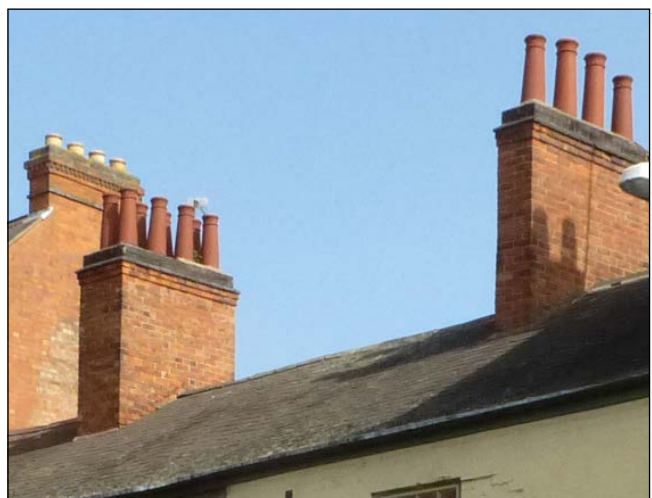
Chimneys and pots on Church Gate.
