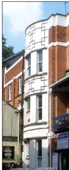
Unusual use of stucco at 66 Church Gate
