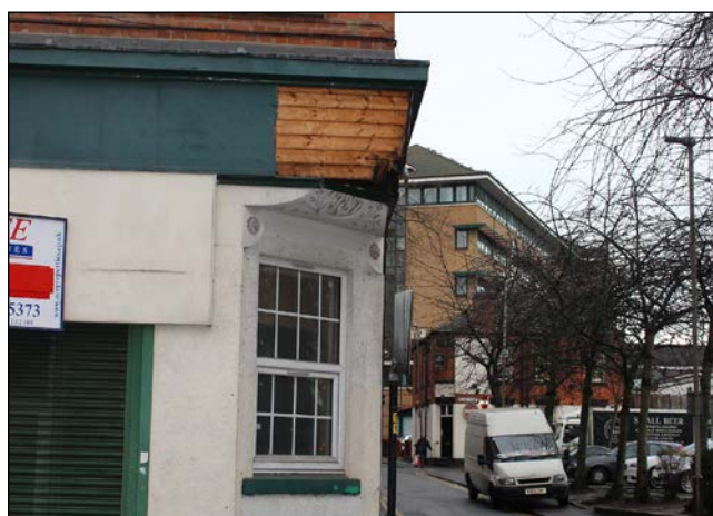
Obscuring of decorative corner feature at 70 Church Gate.
