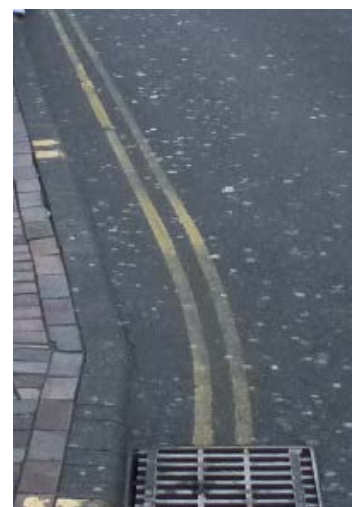
Narrow yellow lines on Church Gate are a way of ensuring correct highway regulations are met while minimising their potentially harmful impact.
