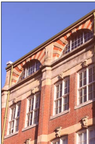
Brick and stonework on 13-21 Church Gate.
