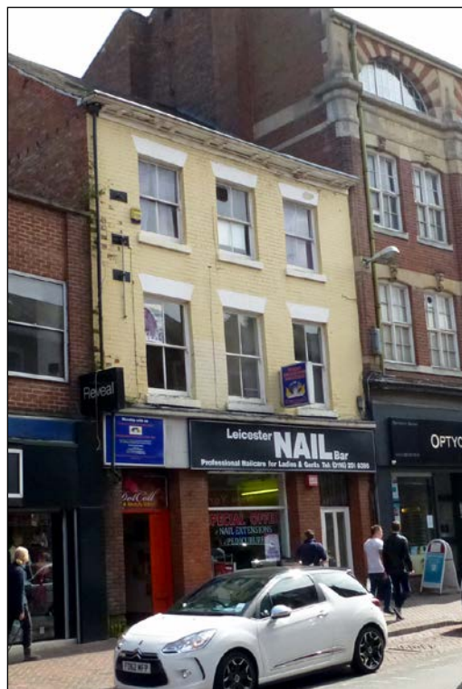
Historic windows that have depth of profile, a traditional opening method and material.
