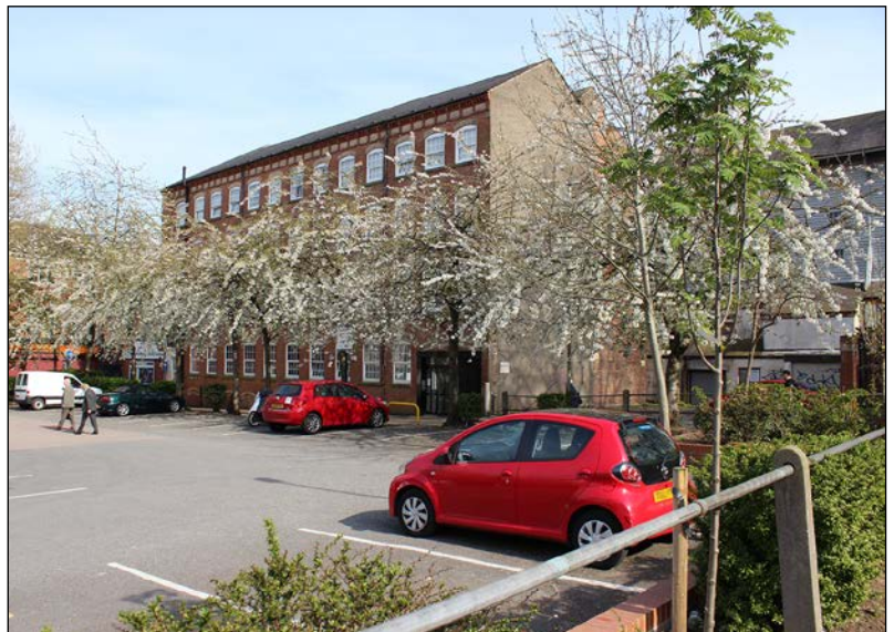
The car park serving Matalan is located on the area thought to formerly be used for Archery Butts. The site has a mixed development history, but is not harmed by being open and contains a large number of trees which make a positive contribution to the area.
