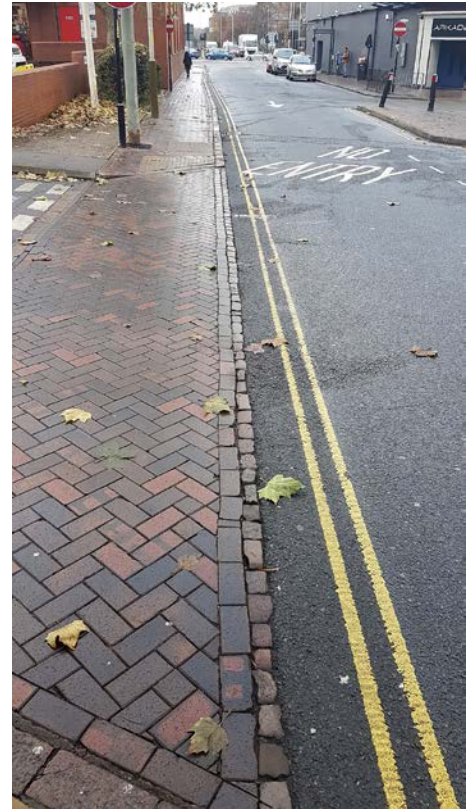
Narrow yellow lines, Church Gate.
