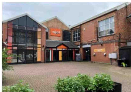
Figure 3: Existing front elevations at 73b Church Gate
