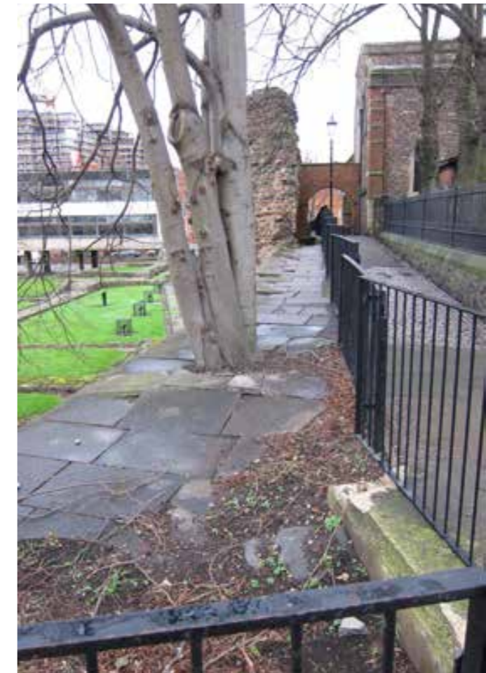
FAR TOP LEFT: EXAMPLE OF CBBLES BEING RE-SET.
